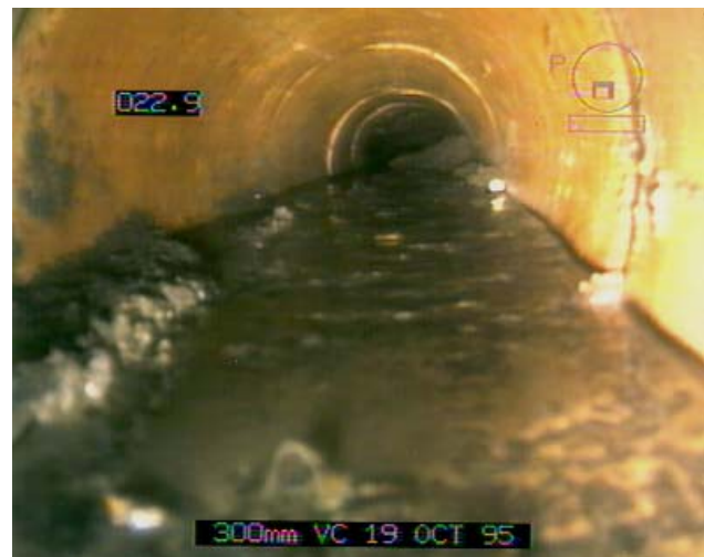
Figure 6: Sedimentation of a stormwater
